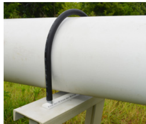
I-Rod® eliminates the crevice by minimizing the contact area and allowing any moisture to evaporate. It's also much easier to inspect.
